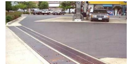
Perimeter Sand Filter
